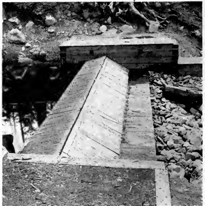
Intake dam and screen chambers at Noon Creek 750 ft. above tidewater.
